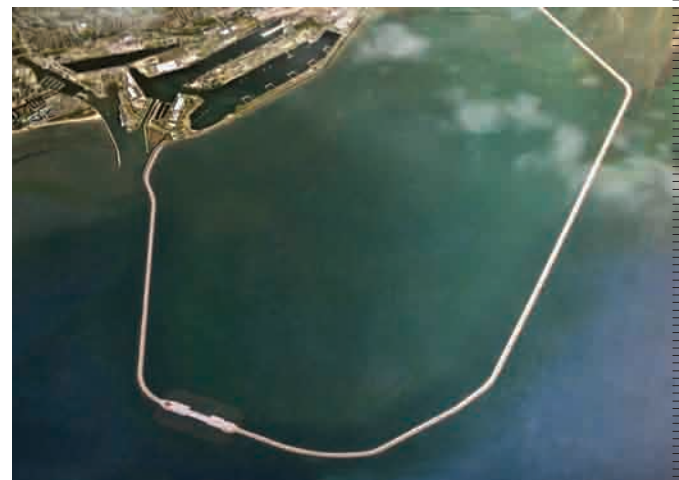
The 9.5 km breakwater will encircle the new 11.5 sq km lagoon in Swansea Bay
