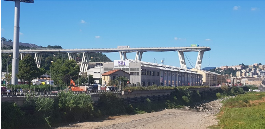
Remains of Polcevera Viaduct
