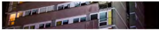
The aftermath of a fire in Belfast which spread via window panels
