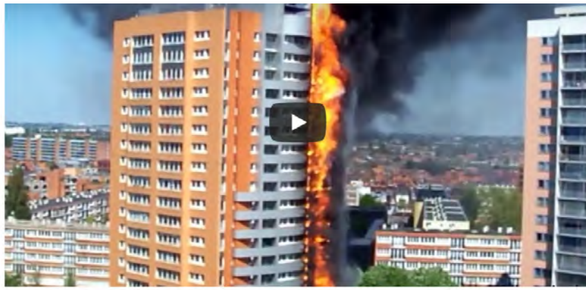
The fire at the Mermoz Tower in France
