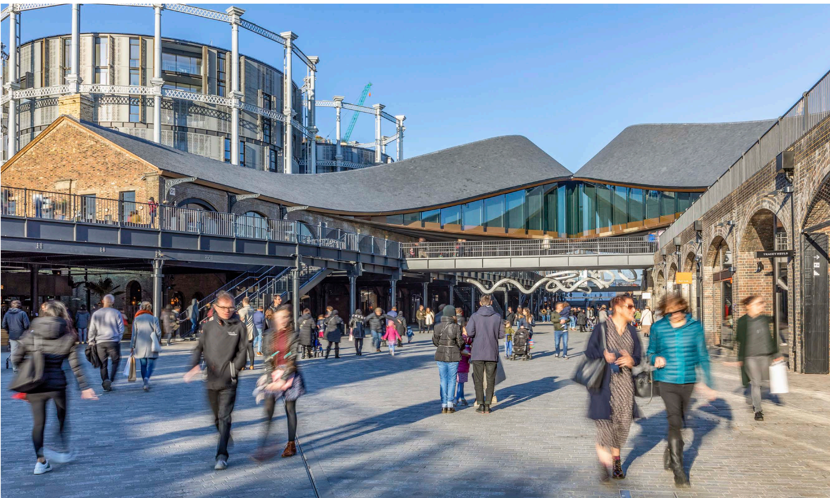
Coal Drops Yard opened in November with a range of high-end shops. The gasworks now contain new luxury flats designed by Wilkinson Eyre
