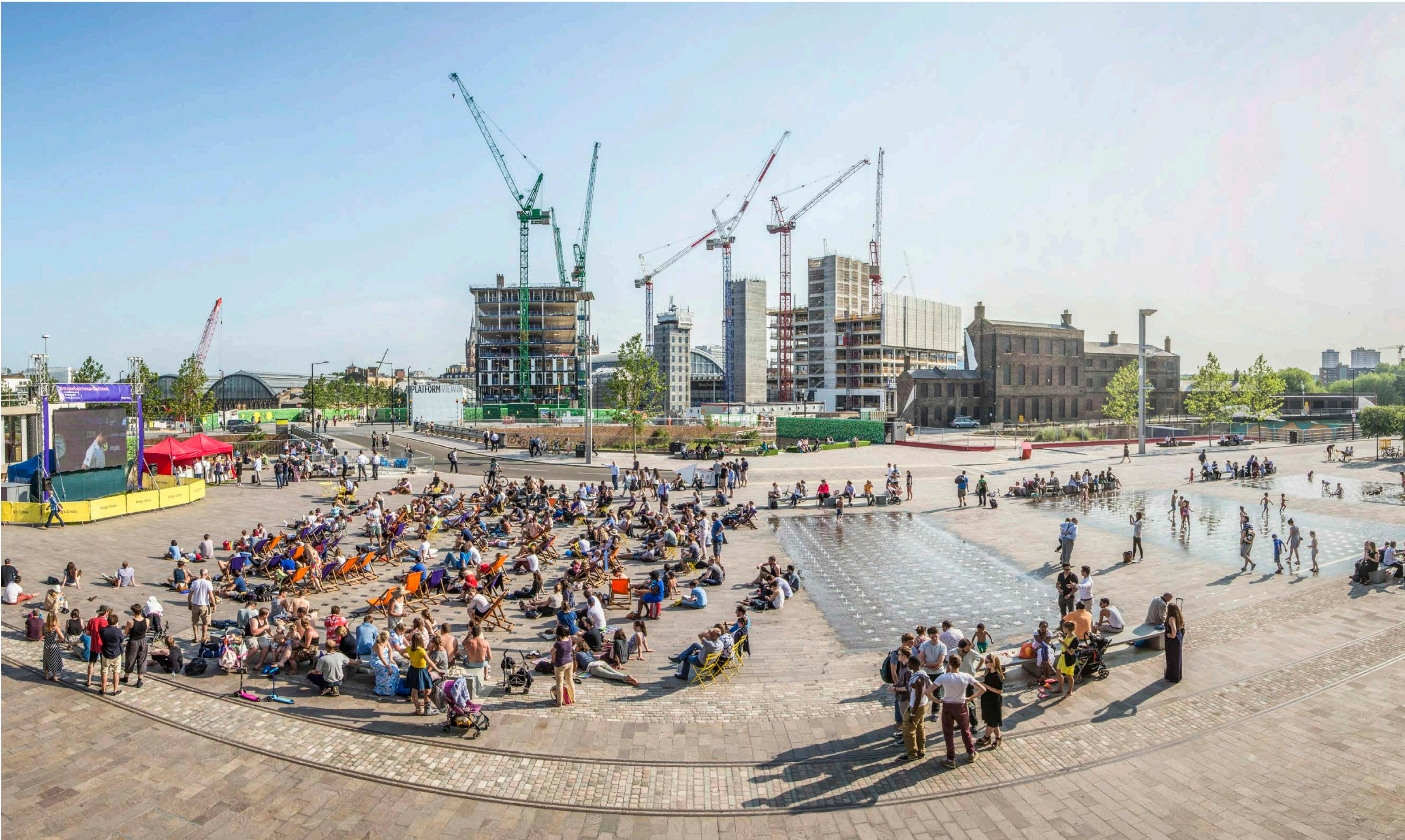
Granary Square has placed public realm at the heart of the development, making what was still a construction site into a destination
