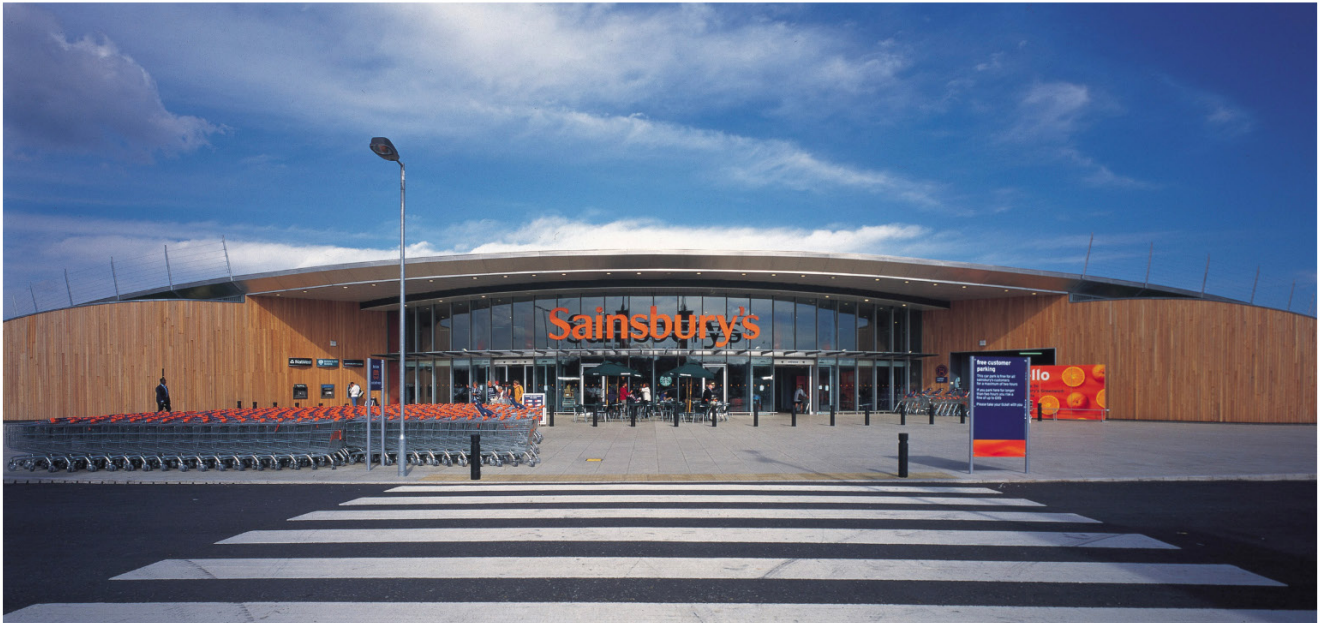
Sainsbury's Greenwich, the UK's most sustainable supermarket, was demolished to build the IKEA store. Photo courtesy of Chetwoods
