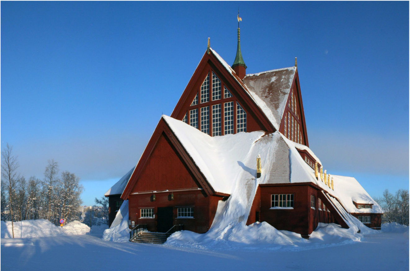
Kiruna's church is being relocated to the new town. Photo is by Heinz-Josef Lucking
