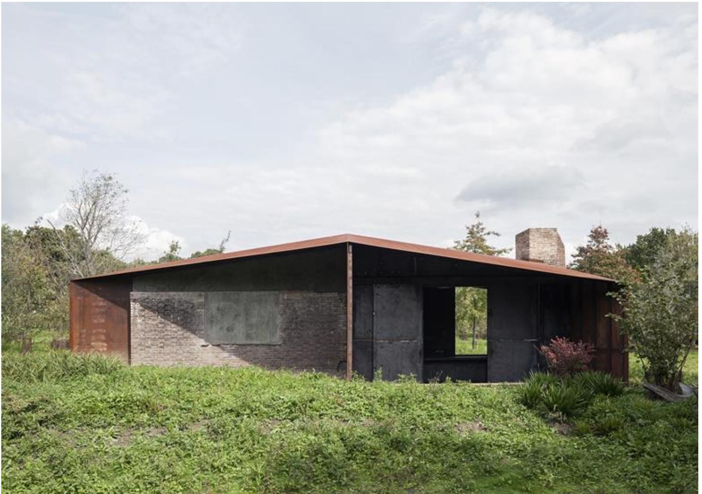
A shallow-pitch corten roof is supported on the concrete walls
