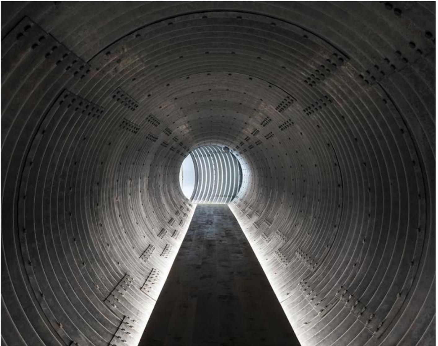
A tunnel encased in a ribbed proprietary tube system links the two buildings
