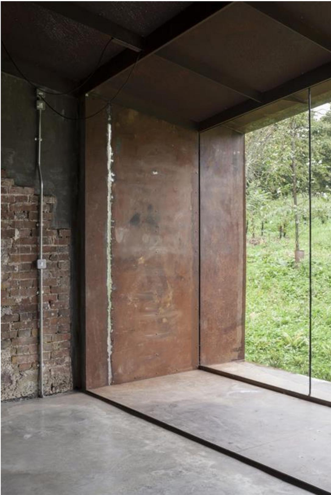
The corten was welded on site and left unfinished with joints and blemishes exposed
